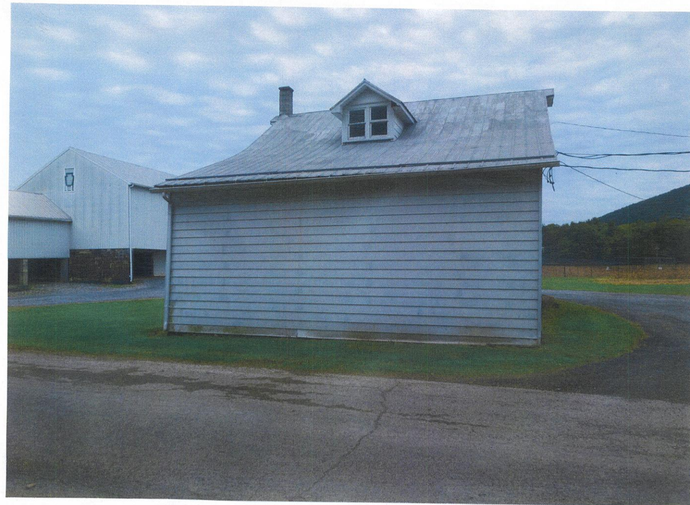
PICTURE OF BUILDING (SOUTH SIDE)
