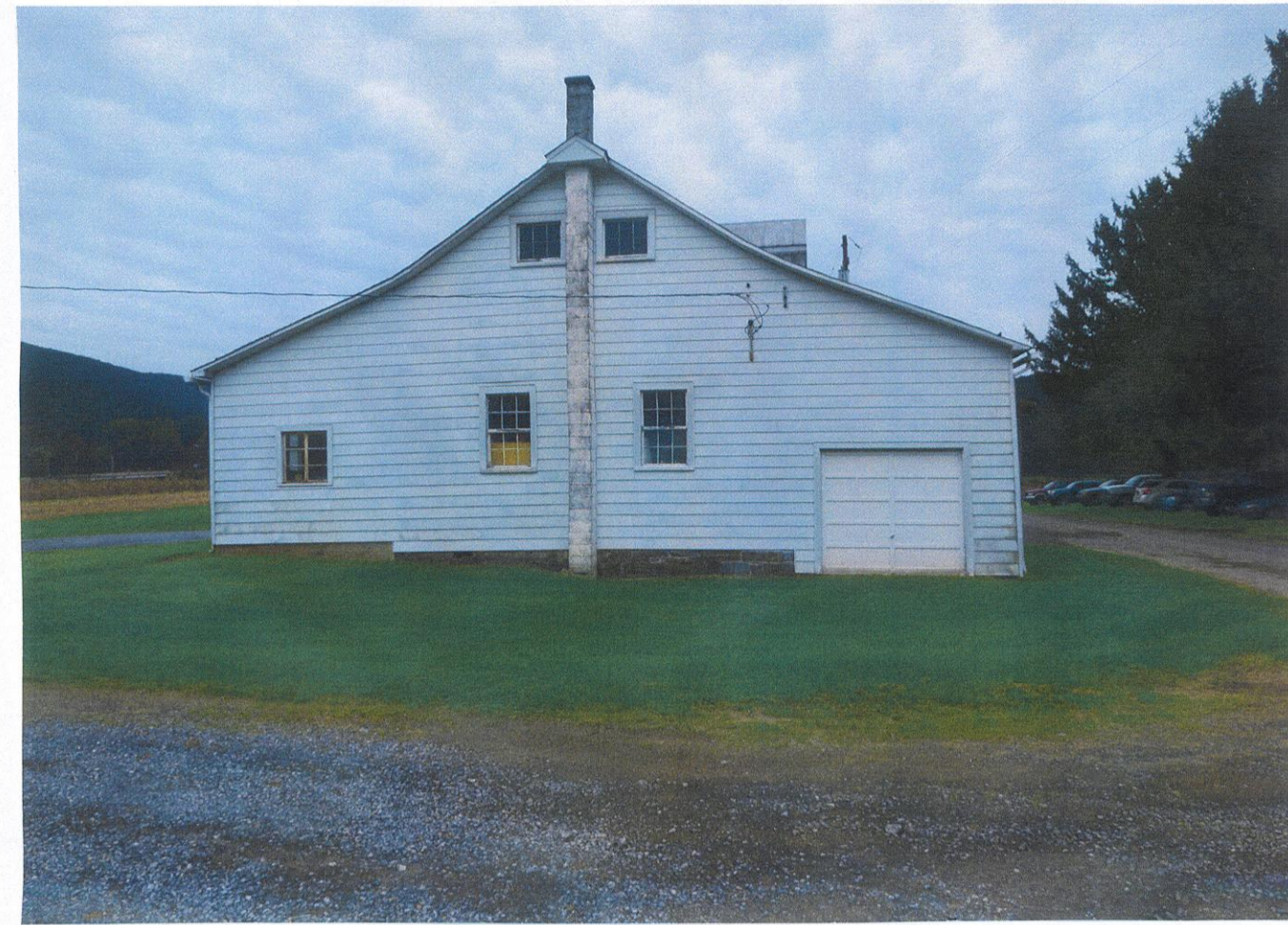
PICTURE OF BUILDING (WEST SIDE)
